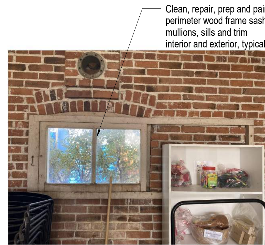
A4 Photo of Existing Conditions (Garage) Not to Scale
