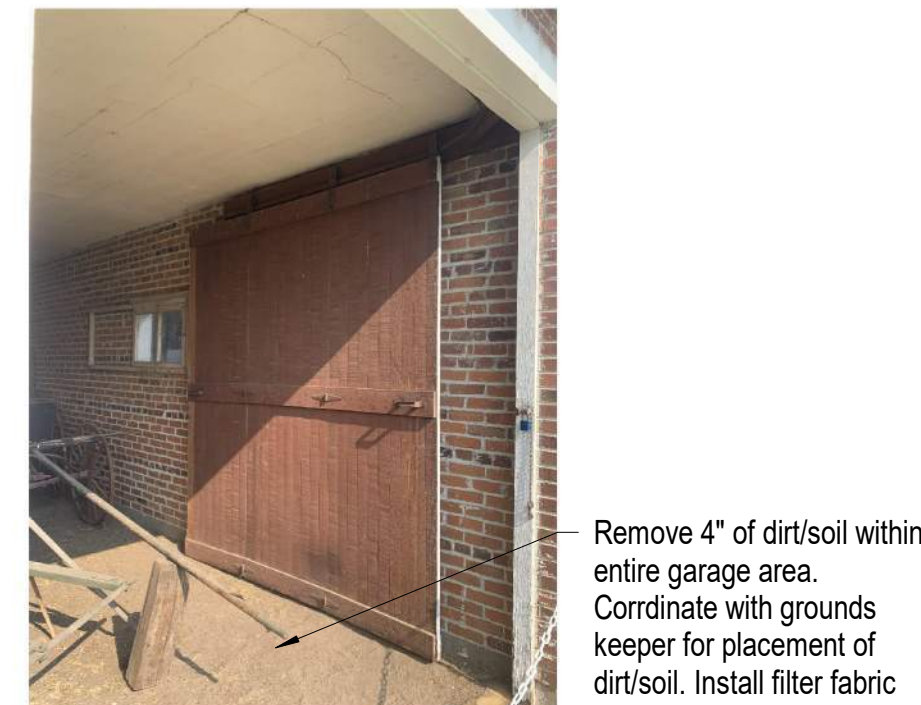
B5 Photo of Existing Conditions (Carriage House) Not to Scale
