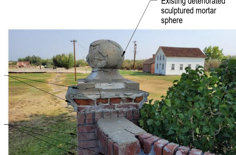
Existing deteriorated sculptured mortar cap Existing lilac bush Existing deteriorated sculptured mortar sphere Existing deteriorated sculptured mortar cap Existing deteriorated sculptured mortar cap Repoint perimeter of deteriorated joints, typical
