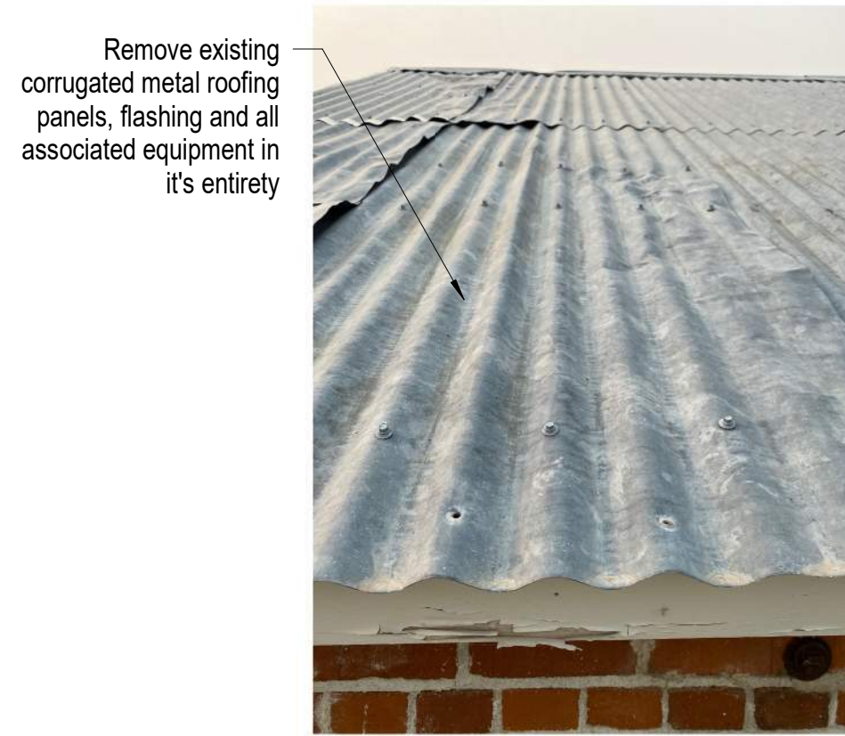
A3 Photo of Existing Conditions (Garage) 12" = 1'-0"
