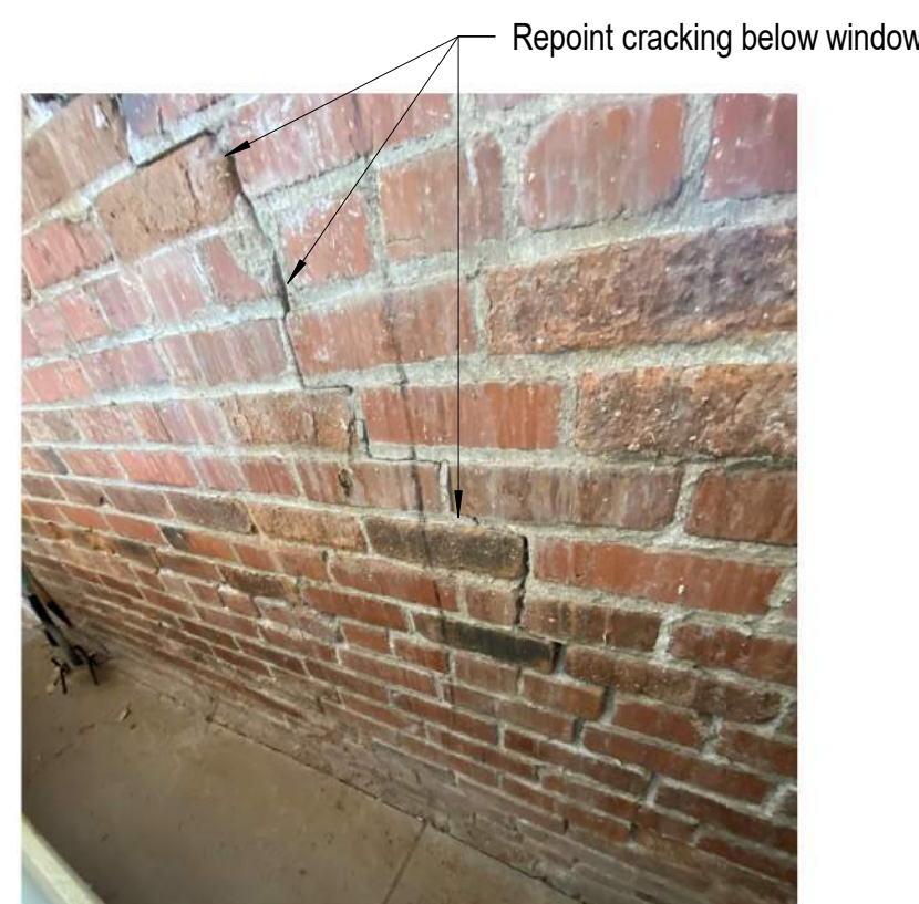
D5 Photo of Existing Conditions (Garage) Not to Scale
