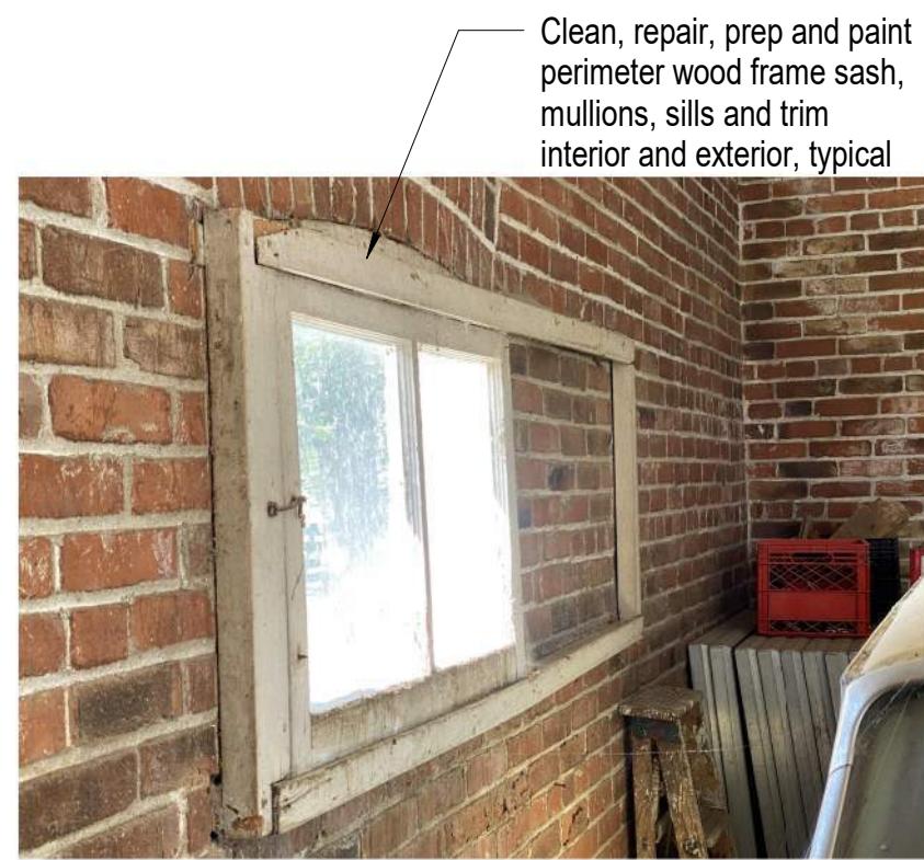
A5 Photo of Existing Conditions (Garage) Not to Scale
