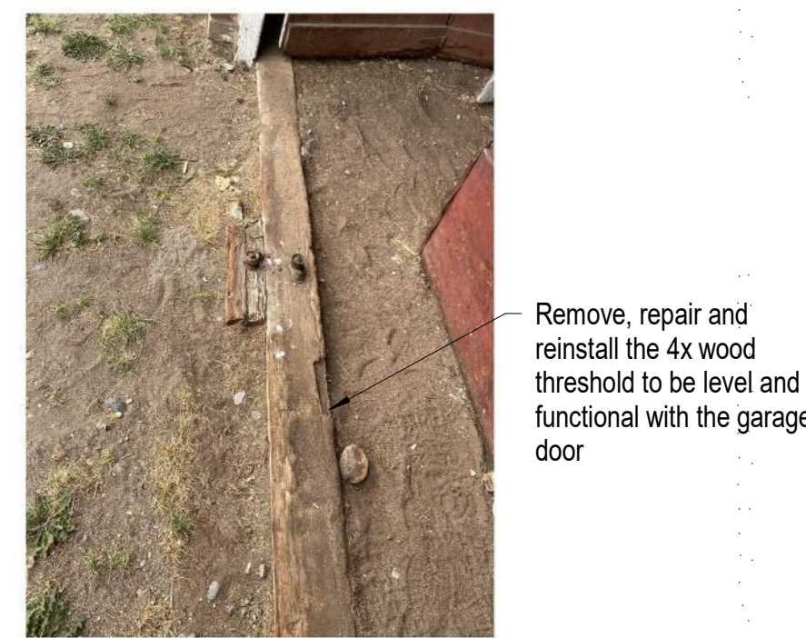
A3 Photo of Existing Conditions (Carriage House) Not to Scale
