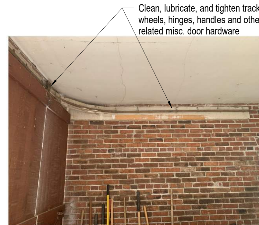
C4 Photo of Existing Conditions (Garage) Not to Scale
