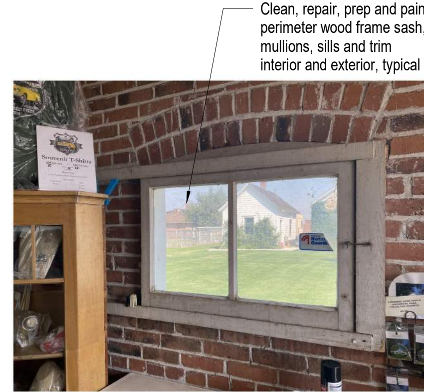
A3 Photo of Existing Conditions (Garage) Not to Scale
