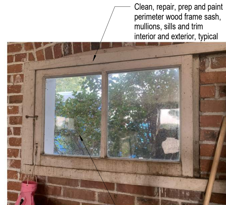
D4 Photo of Existing Conditions (Garage) Not to Scale
