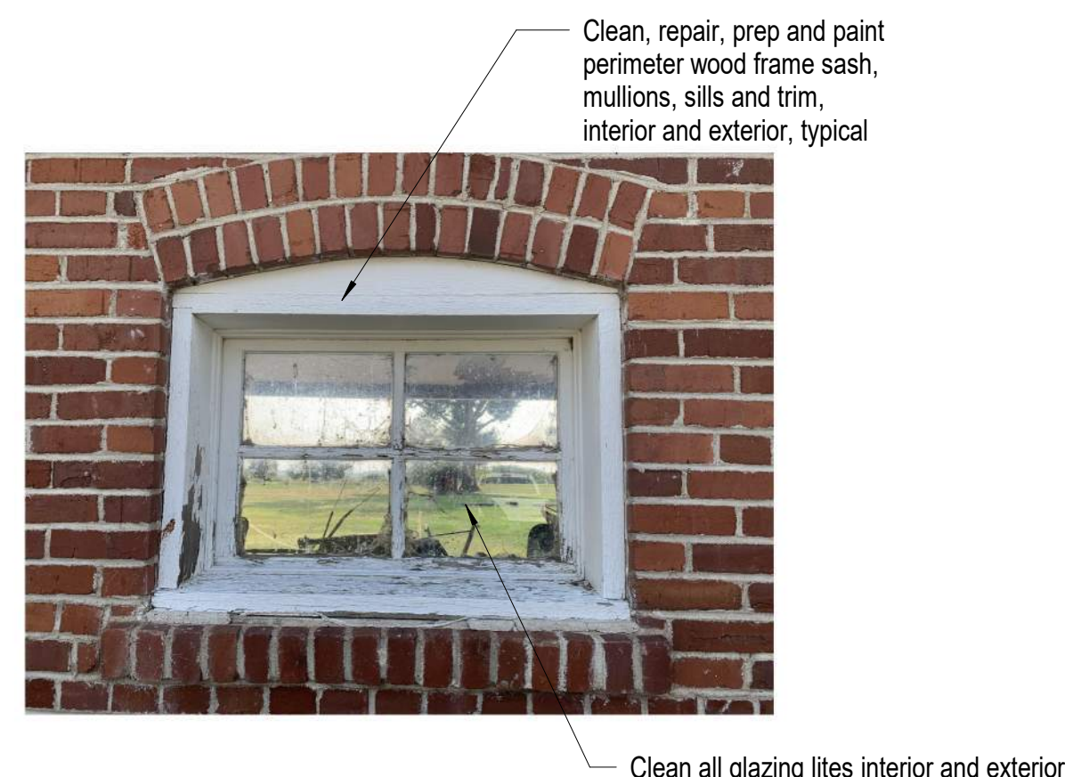
A4 Photo of Existing Conditions (Carriage House) Not to Scale
