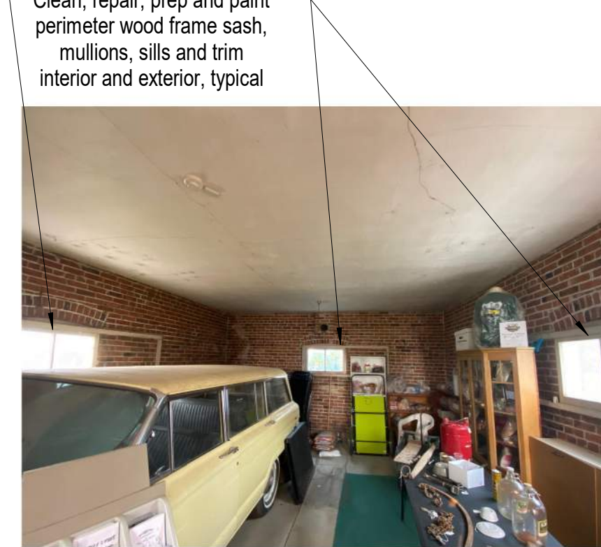
D3 Photo of Existing Conditions (Garage) Not to Scale
