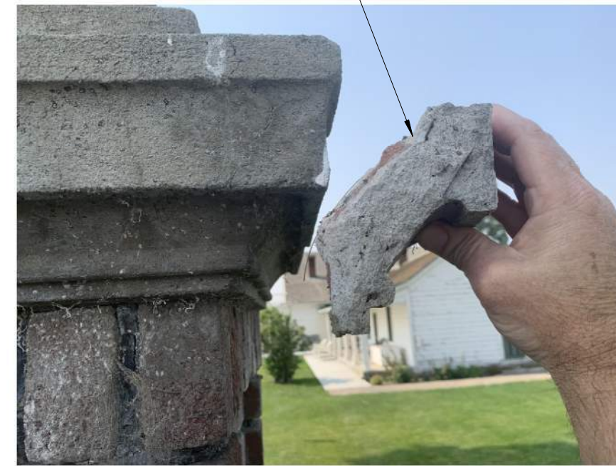
A4 Photo of Existing Conditions (Entry Gateway) Not to Scale
