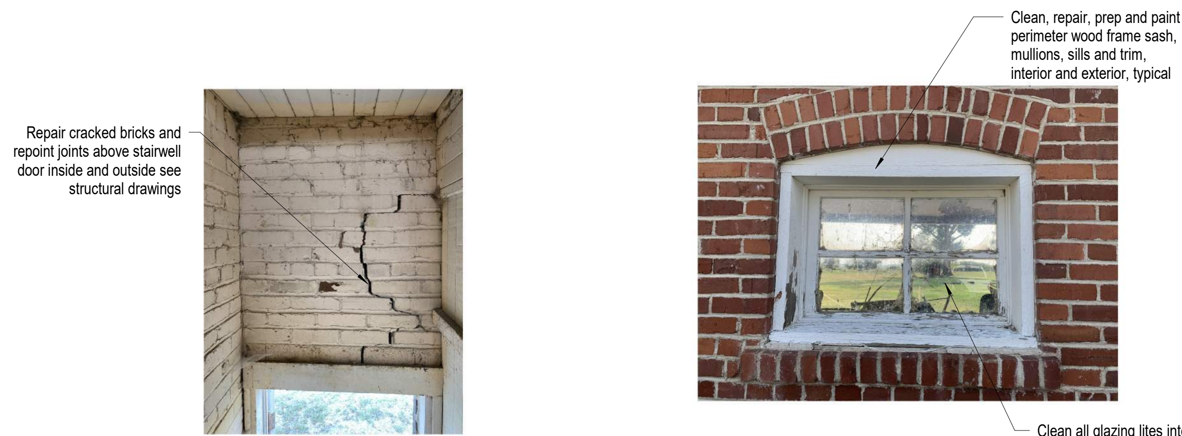
A5 Photo of Existing Conditions (Carriage House) Not to Scale
