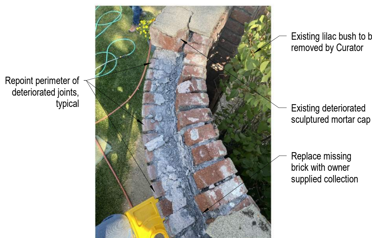
D5 Photo of Existing Conditions (Entry Gateway) Not to Scale
