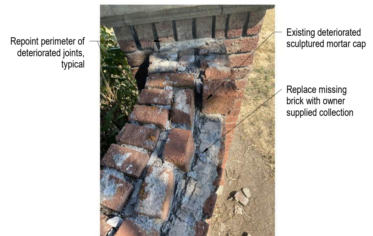
C5 Photo of Existing Conditions (Entry Gateway) Not to Scale
