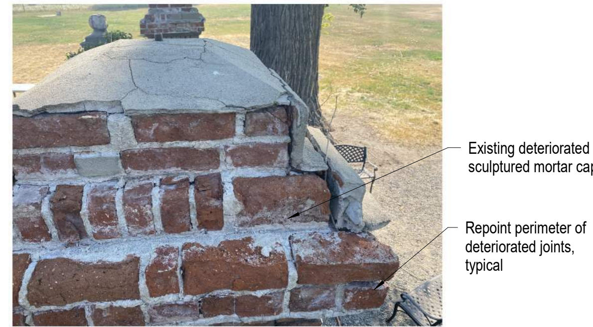
A5 Photo of Existing Conditions (Entry Gateway) Not to Scale
